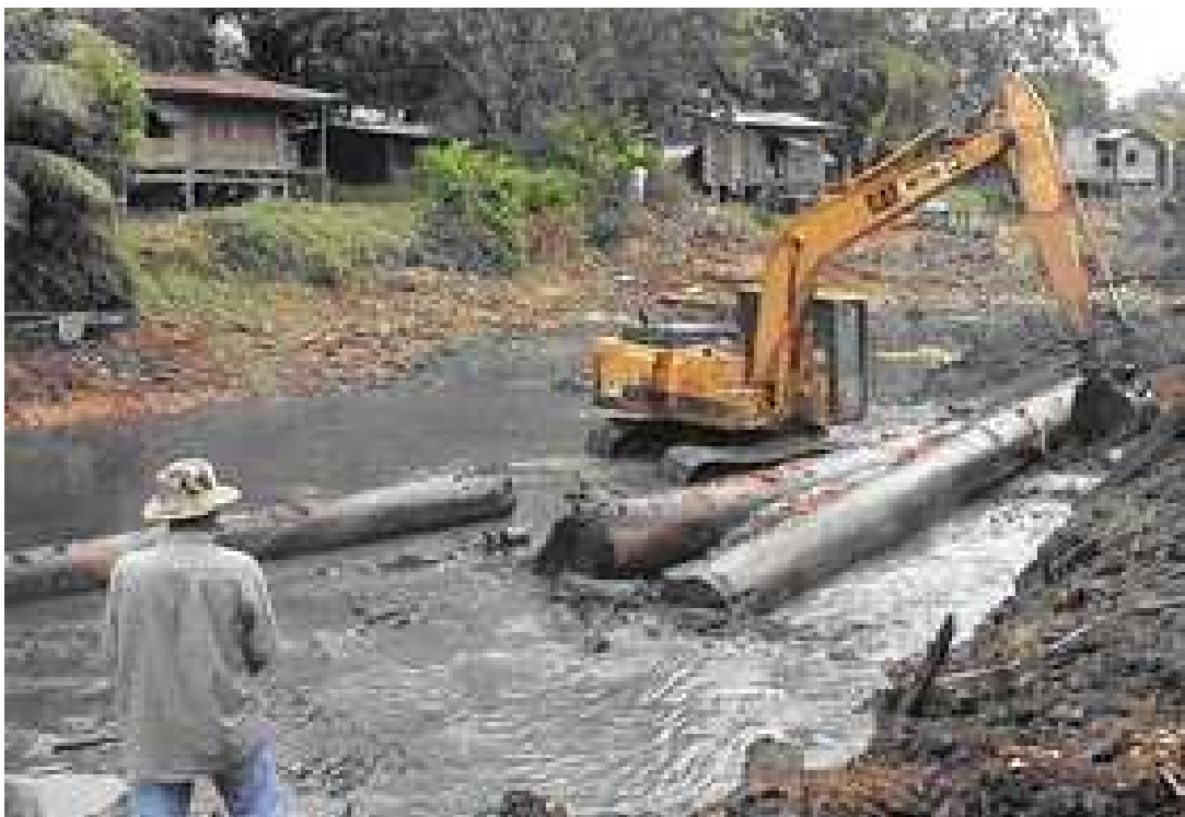
Figure 23 The river is being dredged
