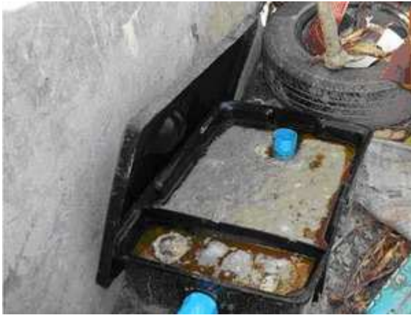
Figure 17 A grease trap outside of a house
