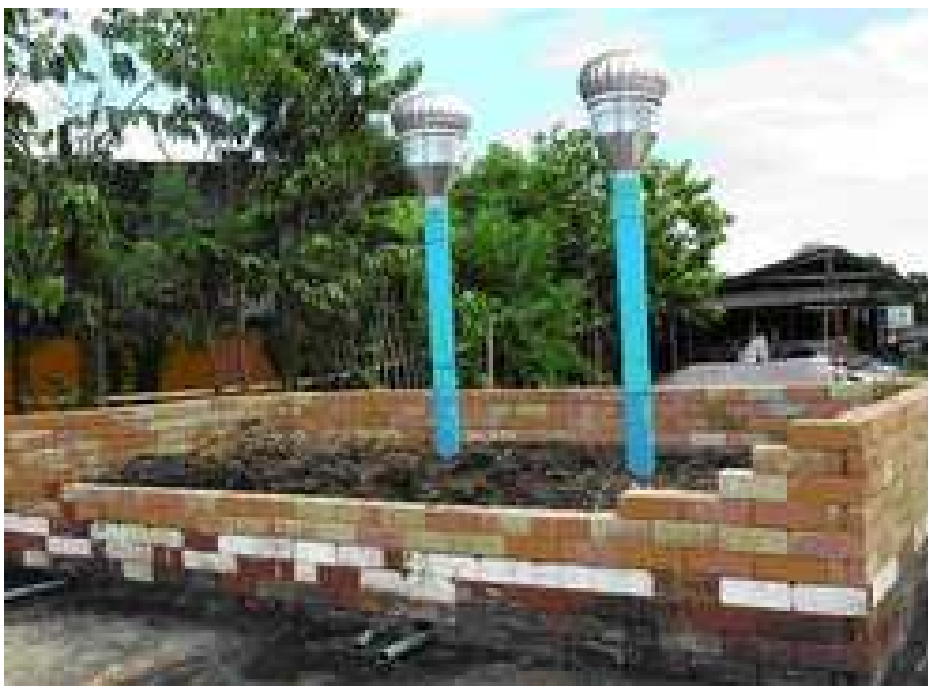
Figure 29 A compost production pit with ventilator and drainage ducts
