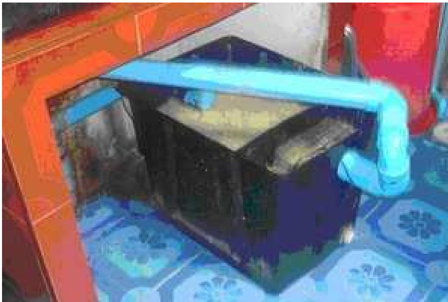
Figure 16 Grease trap installed under a washing sink
